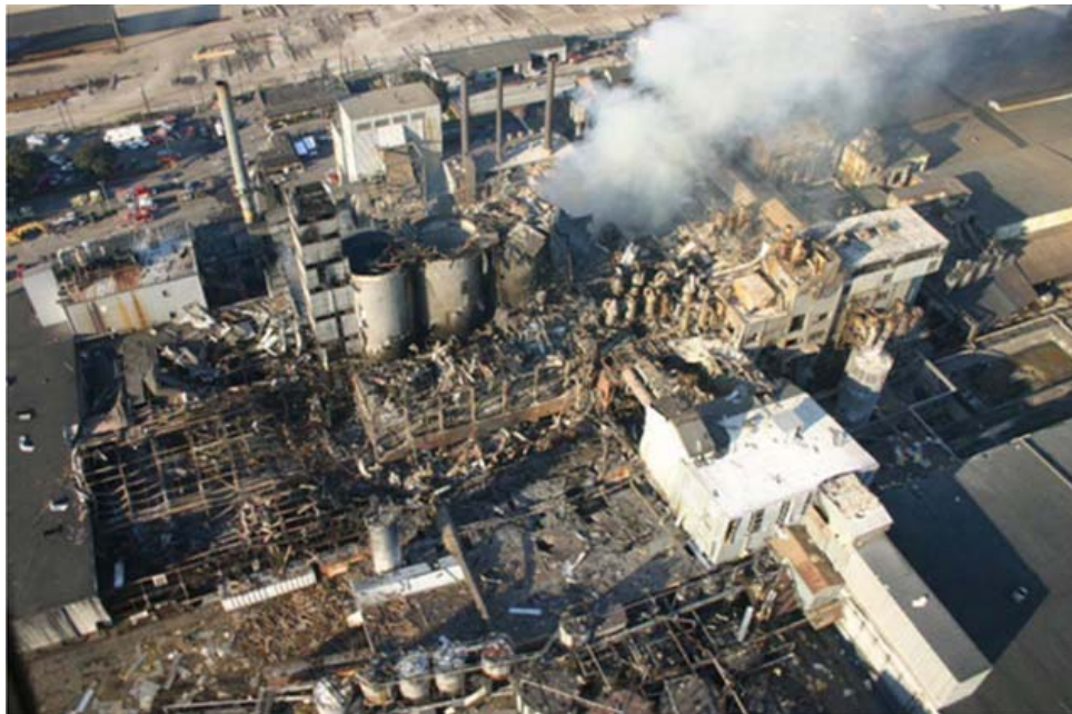
Figure 5: Sugar Dust and Explosion Fire Accident, Port Wentworth, Georgia 7
