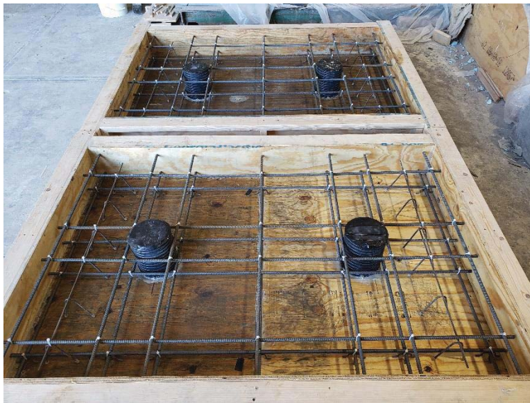
Figure 4.032: Shear Pockets Forming and Slab Reinforcement Details.
