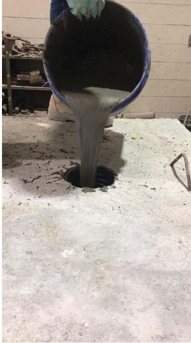
Figure 4.035: UHPC Casting for UHPC#2 Specimen.
