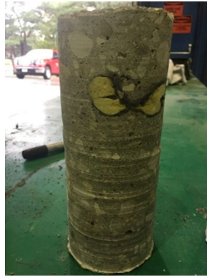
Figure 2.18 Slab 3 - Core 12 (Oblong Void)
