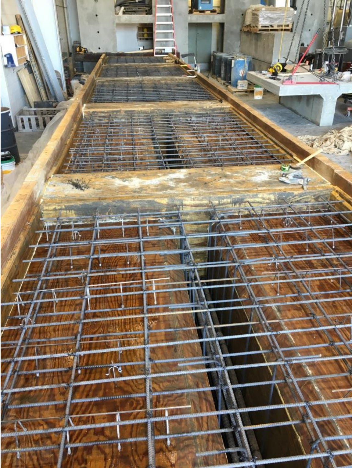
Figure 4.9: Steel Assembly for the Second Pour
