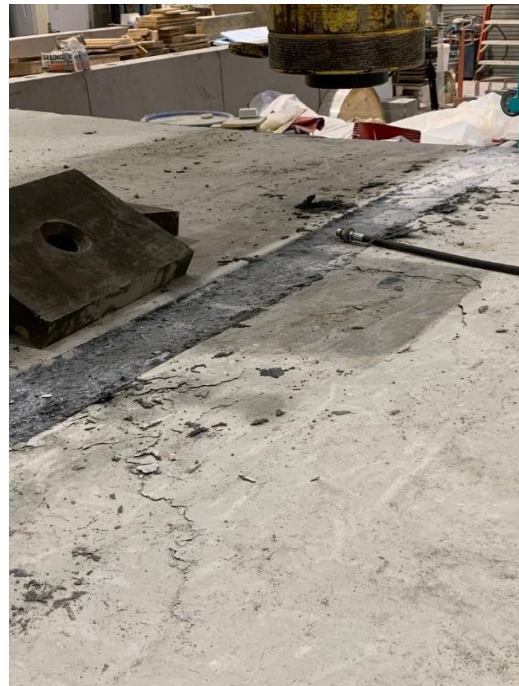
(b) After failure
