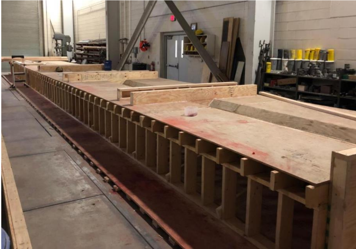
Figure 4.3: Full-Scale Formwork Assembly
