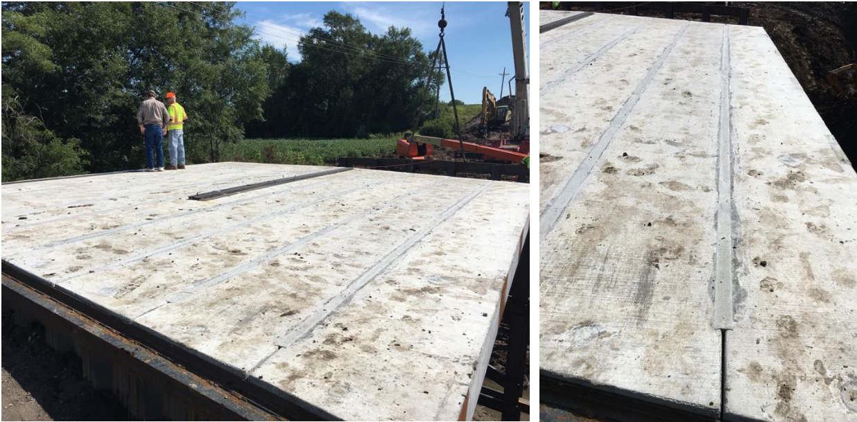
Figure 1.3: Grouts Between Longitudinal Shear Keys
