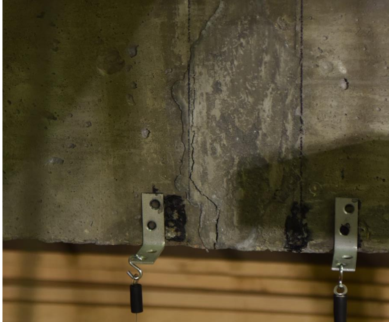
Figure 3.12: Initial Cracking at the Grout Interface (Specimen F-F-1)
