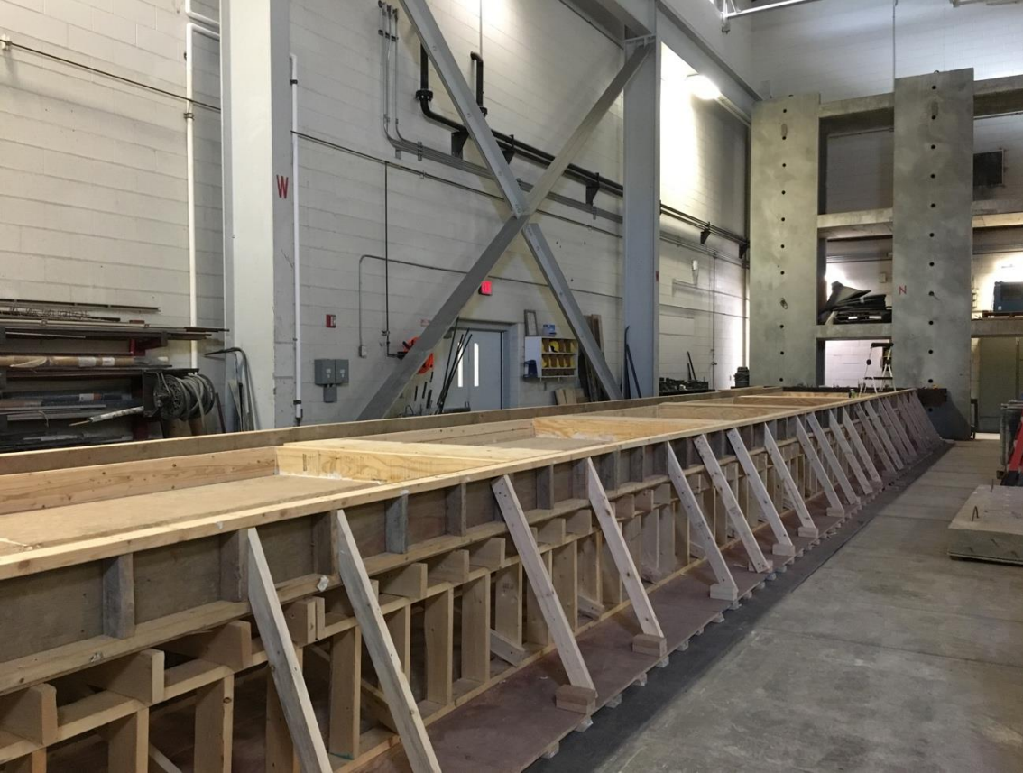
Figure 4.4: Complete Full-Scale Formwork for County Bridge Specimen
