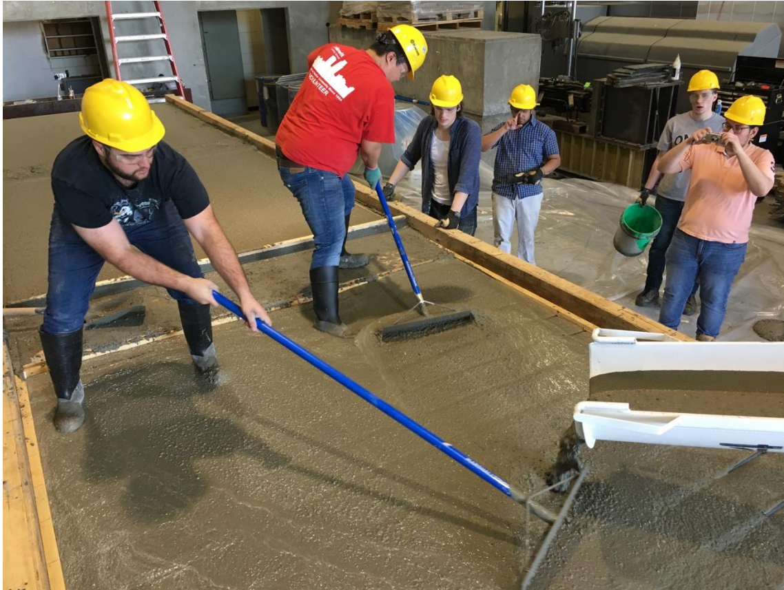
Figure 4.7: Casting Self-Consolidating Concrete for Full-Scale Bridge Specimens
