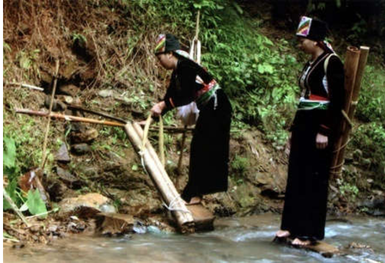
Figure 5.9: Current potable water system in remote areas of ethnic minority group in Son La province
