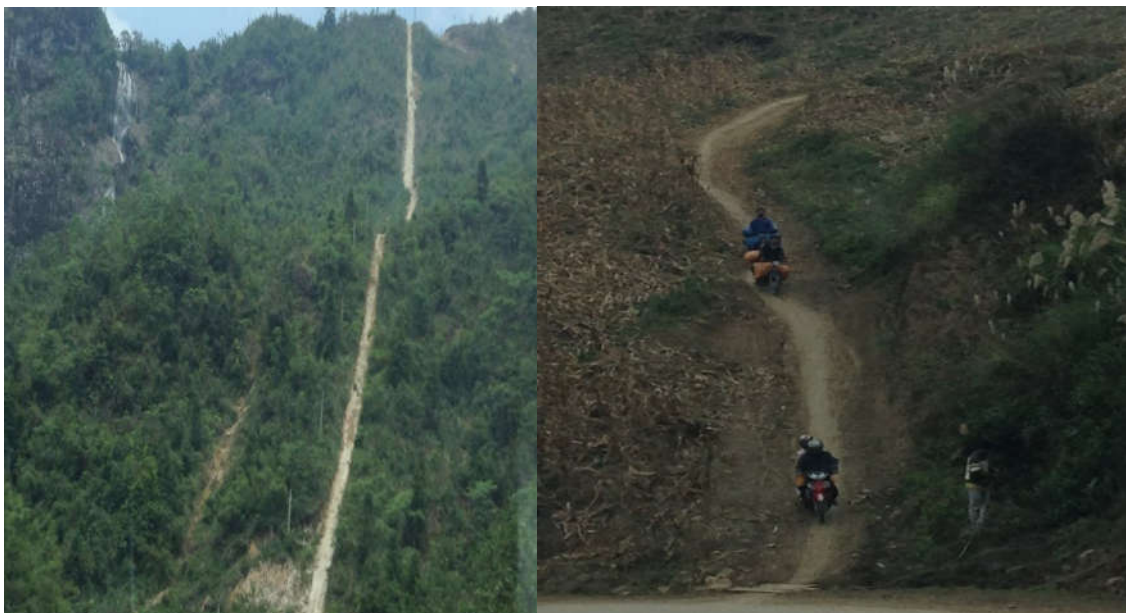
Figure 5.6 : The road connecting commune of H'Mong group to national road in Bac Yen district
