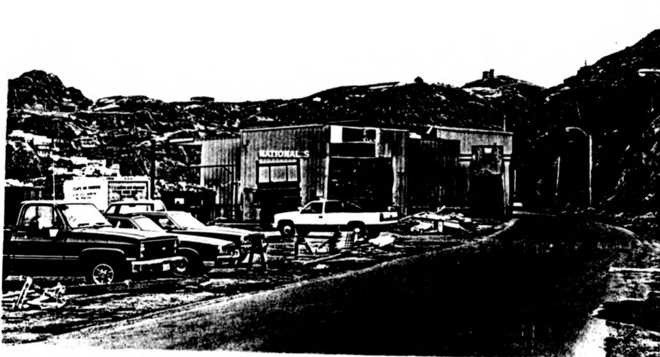
Picture: National Sea Plant in St. John's Being Torn Down. April 1996.
