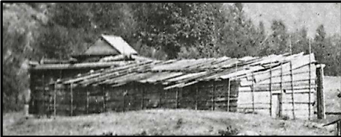
Figure 2.2. A Coast Salish single pitch plank house at Comiaken Village on the Cowichan River in 1869. (Dally 1869).
