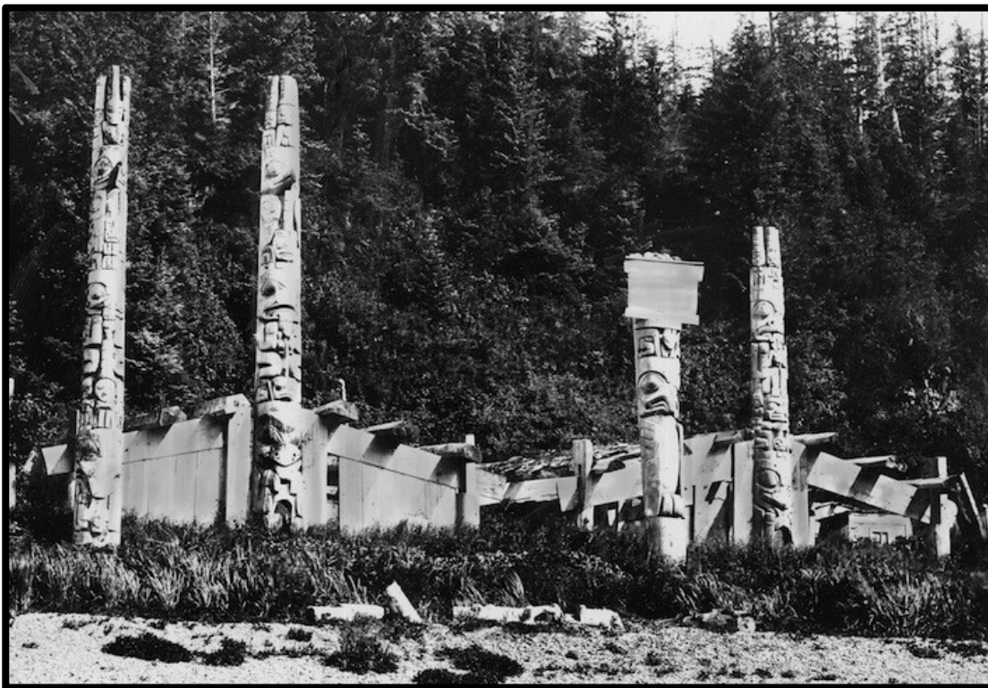
Figure 2.5. Six beam gable roof cedar plank houses at the Haida village of Cumshewa (Dawson 1878).
