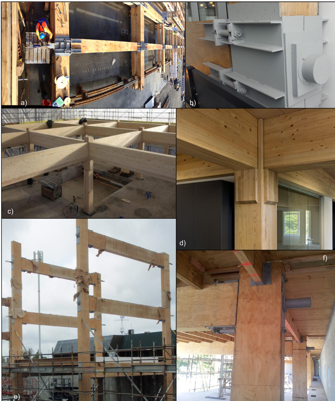
Figure 1. Examples of operative PresLam structures and beam-column joint detailing: a) Trimble Navigation Offices, Christchurch (courtesy of Paul Drummond) using b) external steel plates in the beam column joint; c) ETH House of Natural Resources, Zurich (copyright ETH Zurich-Marco Carocari) using d) hardwood columns (copyright ETH Zurich-Marco Carocari); e) Merritt Building, Christchurch (courtesy of Andy Buchanan) using f) internal steel plates (courtesy of Andy Buchanan).
