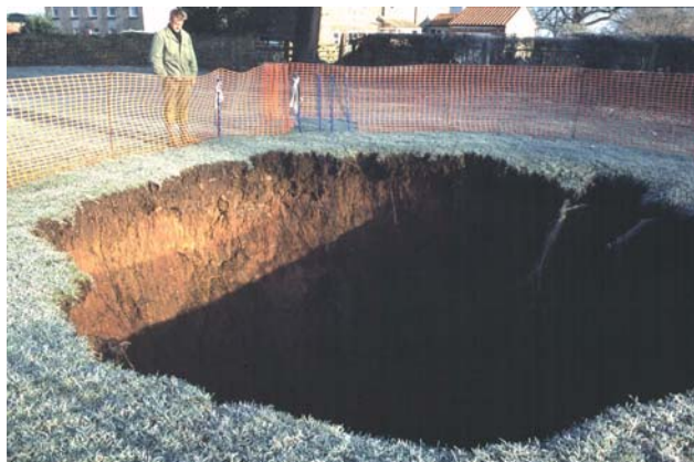
Figure 2. Subsidence crater (doline) caused by the dissolution of Permian gypsum beneath the village of Sutton Howgrave, North Yorkshire [SE 3146 7928]. The hole started to collapse in December 2000, the photograph was taken on 14 th February 2001 when the hole was 5-6m in diameter and 11m deep with water at a depth of 8m. The crater is about 400m from the gas pipeline. Photo A.H.Cooper © NERC.
