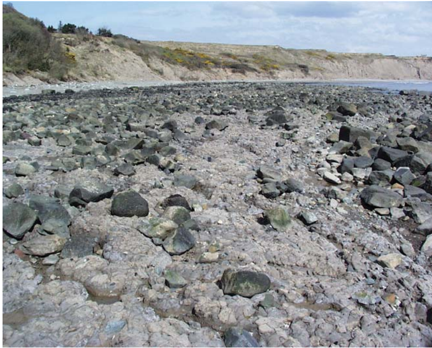
Figure 11. Remnants of light brown to purple stiff fissured clay on the foreshore in front of Treheli at which is probably the remnants of toe heave resulting from a deep-seated rotational landslide.
