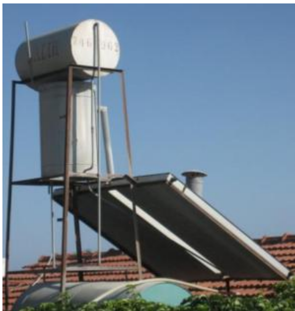
Figure 2.2: Pressure-Less Thermosyphon System with Vertical Hot Water Storage and Horizontal Supply Tank in Turkey
