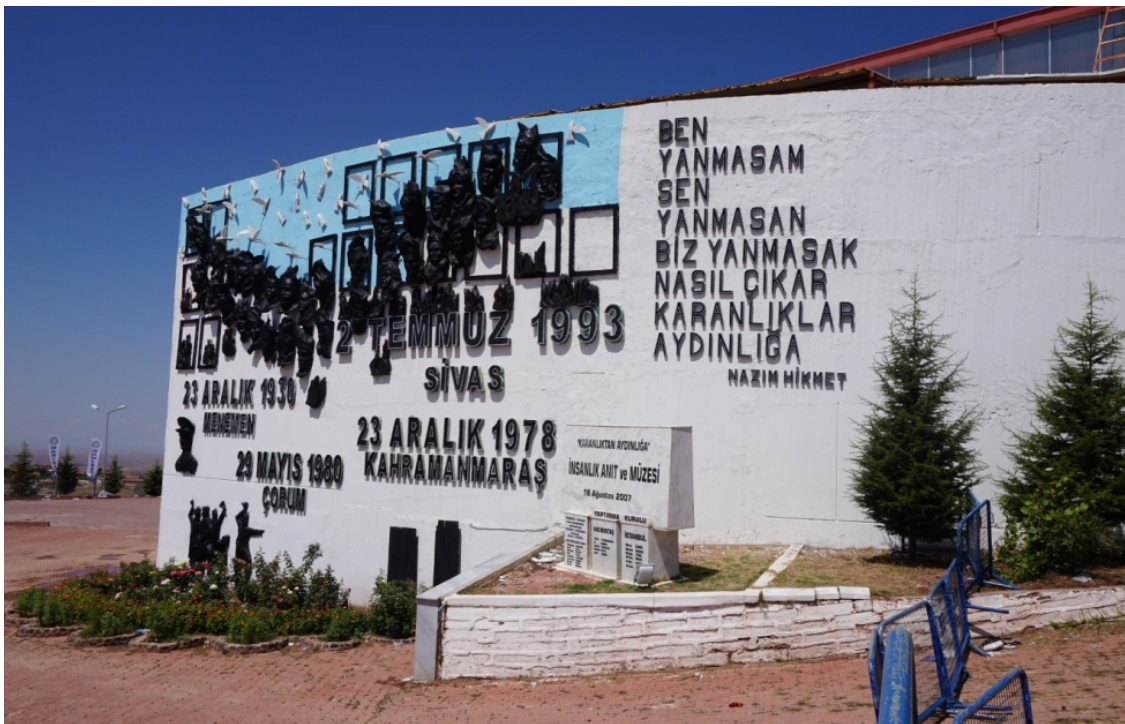
Figure 3. Wall of a building recently erected in Hacibektaş. Photo by Sinibaldo De Rosa, August 2015.
