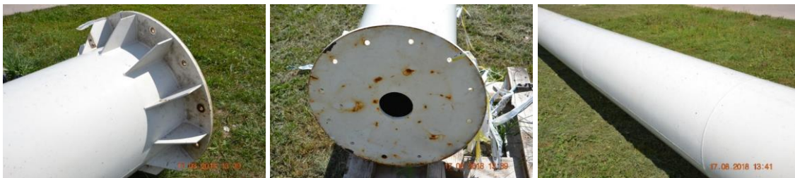
327 Figure 6. Views of the VAWT parts: bottom platform of the foundation (left), top platform (centre), welding 328 lines between two segments and along two parts of one segment (right)
