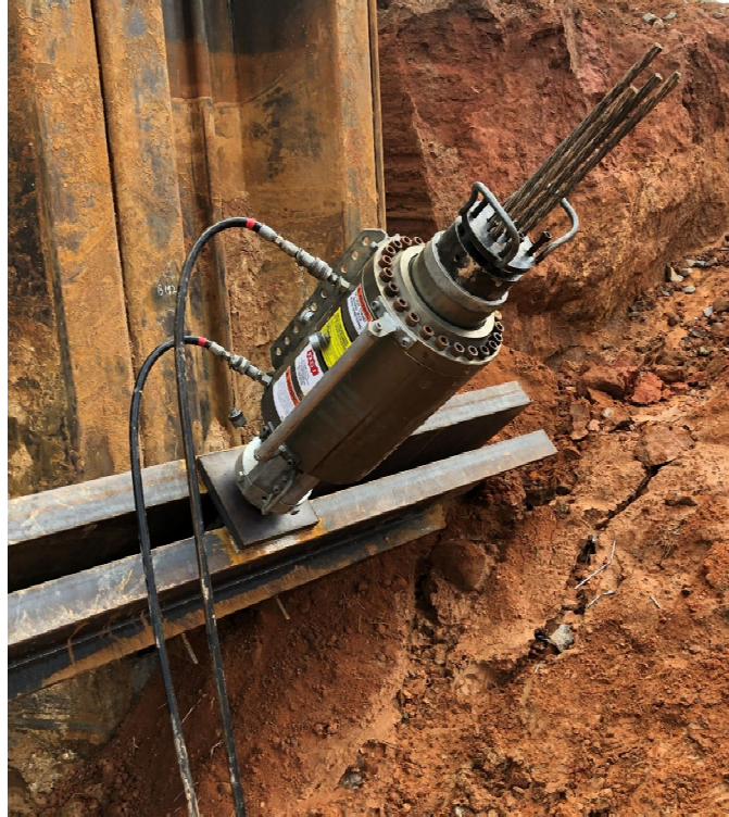
Figure 11-3. Tensioning of 4-strand tieback anchor with hydraulic jack.
