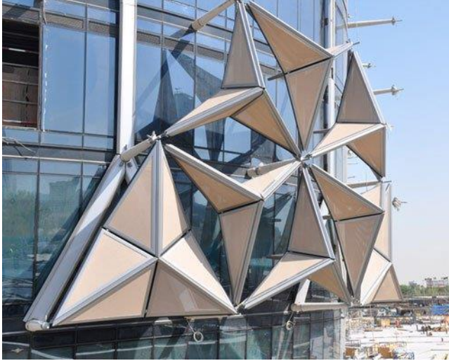
Figure 42: Installation of Mashrabiya Screens
