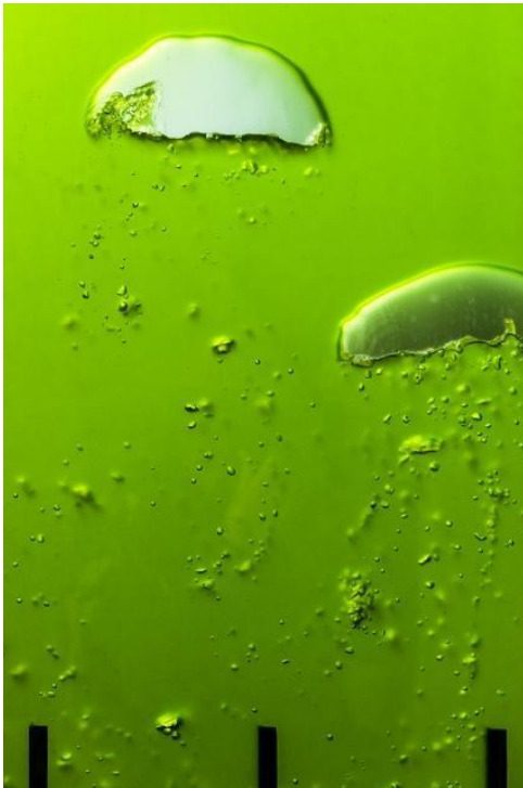
Figure 48: Microalgae infused glazing panels: SolarLeaf
