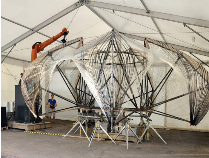
Figure 11: Robotic arm fabricating ICD/ITKE Research Pavilion, Stuttgart, Germany, 2012
