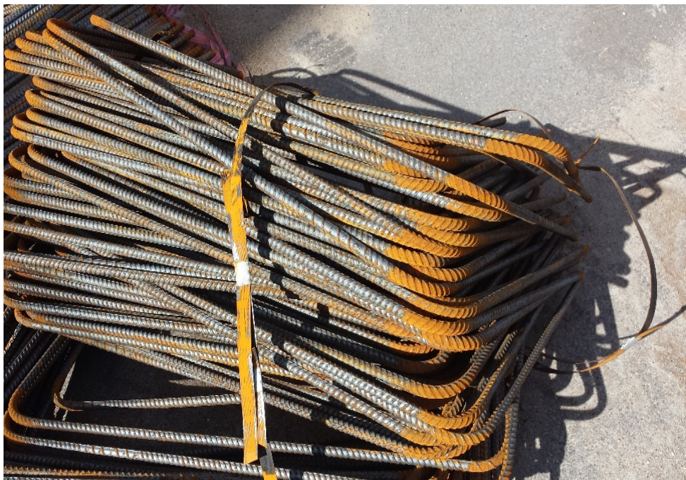
Figure 4-1. Accelerated general corrosion in the area of bending.
