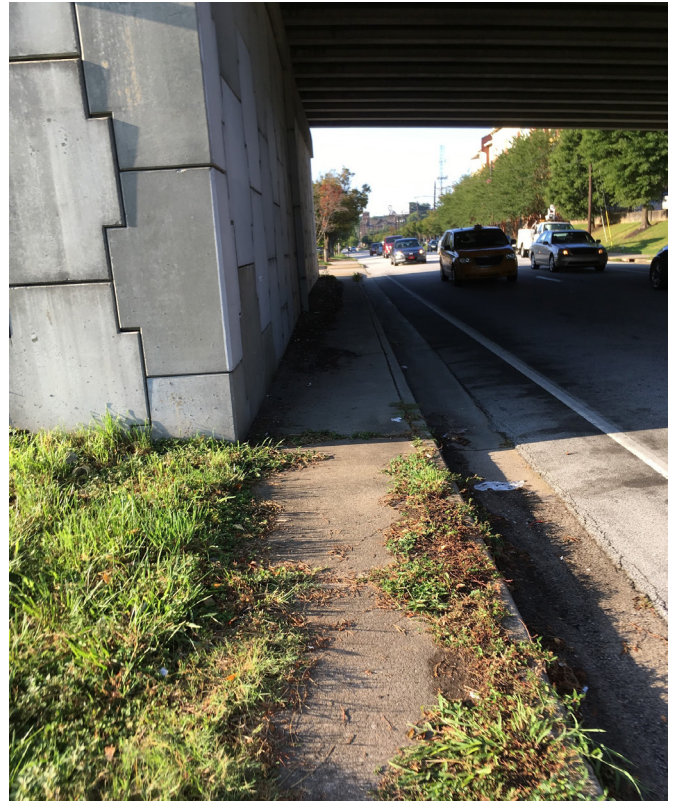
Figure 58: Central Avenue Underpass (Andreas Wolfe)
