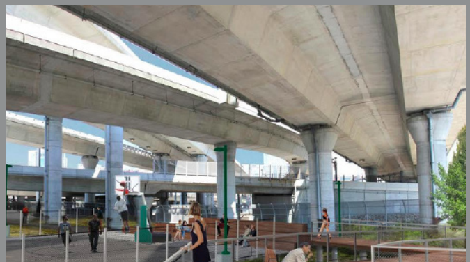
Image source: MassDOT
