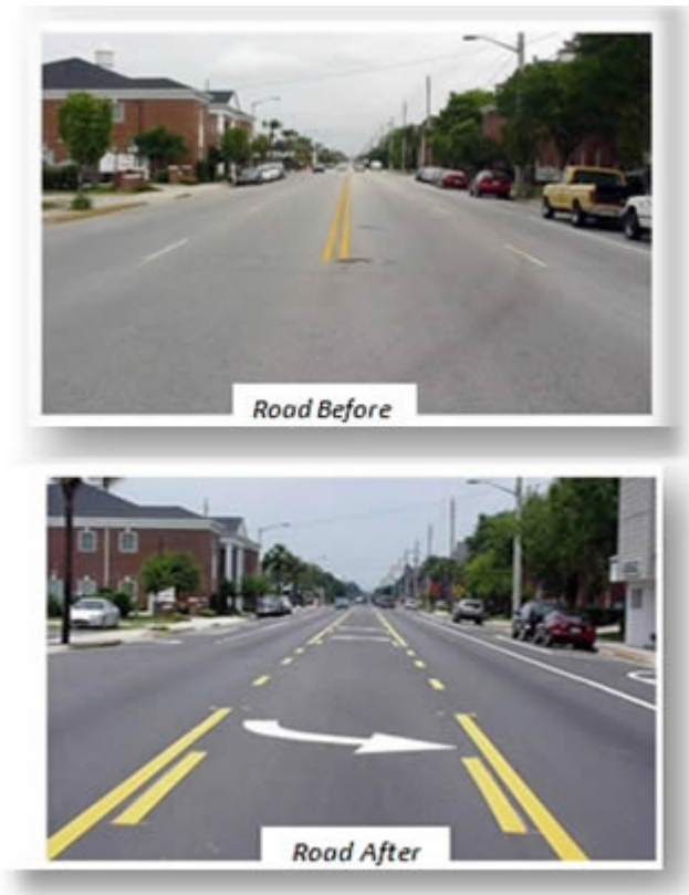
Figure 54: Example of a road diet or lane re-configuration to allow for bicycle lanes ( Federal Highway Administration )
