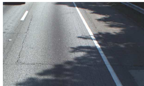
Figure 2-8 – Examples of cracking on I-285 in 2013 (left) and 2017 (right)
