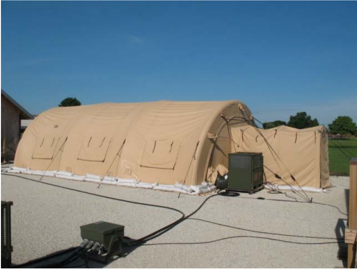
Figure 12 – Airbeam Shelter Perspective View 1: L×W×H = 20 ft × 32 ft × 11 ft [42]
