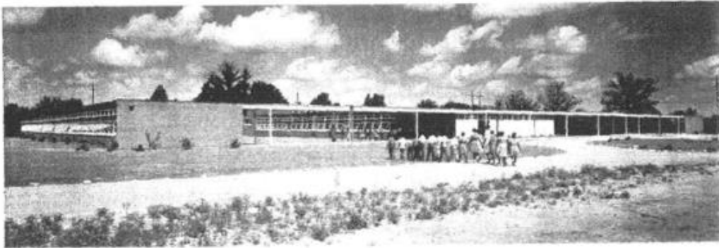
Illustration 26. Plan and photograph of McCoy Hill School in Americus, a small town in south Georgia. Designed by Stevens and Wilkinson, and part of the “separate but equal” efforts of Georgia to avoid integration, this school was built for African-American children in 1956. Apparently the school housed both primary and secondary students as the wing on the south is labeled “primary classrooms.” Pictures and plan from Selected Works of Stevens and Wilkinson , pp. 104-107.
