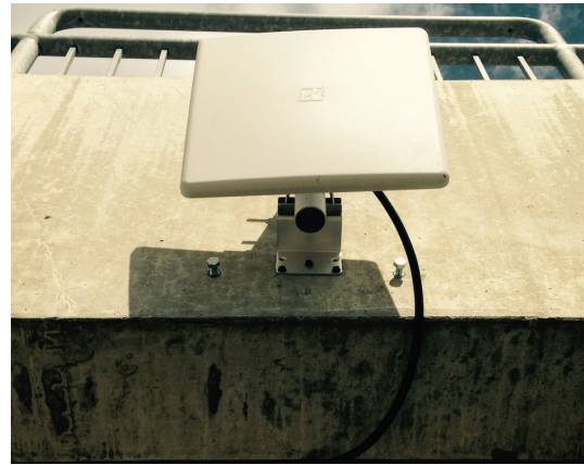
(b) RFSN1 2.4/5GHz antenna mounted in the stadium
