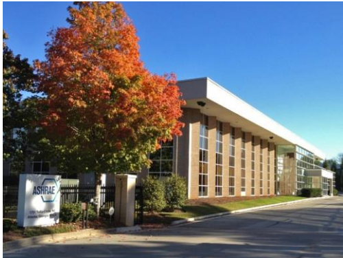
ASHRAE Headquarters with Geothermal Heat Pump
