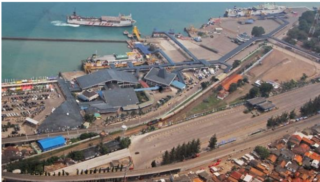
Figure 2.3 Ferry port authority Merak
