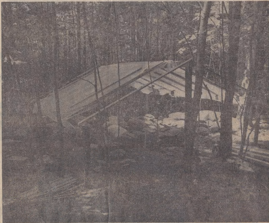
A plastic cover protects workers at the burial site.
