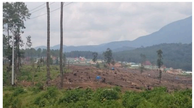
Fig. 8. Siosar relocation village and surrounding reclaimed pine forest.
