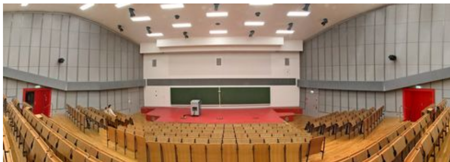
Figure 4.11.: Photo of the WFS loudspeaker system in an auditorium of the Technische Universität Berlin with 832 channels and more than 2700 loudspeakers. ©Pressestelle der TU Berlin, taken from Technical University Berlin (2015).
