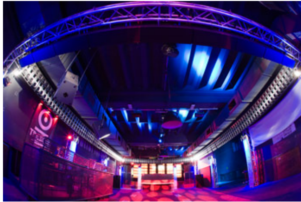
Figure 4.10.: Photo of the IOSONO WFS loudspeaker system in the Tresor club Berlin. The speakers used to be arranged above the audience surrounding the dance floor. From IOSONO GmbH (2008).
