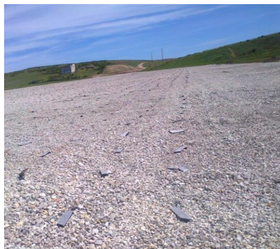
Figure 2. Installed vertical drains before embankment 3119
