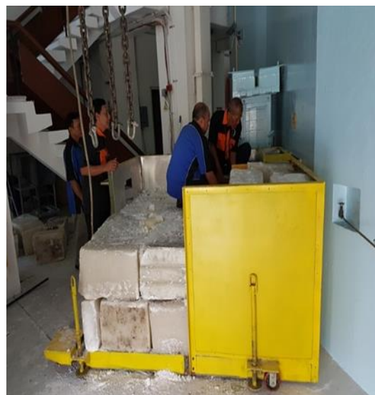
Fig 7. Revitalization of paraffin shielding placed in cubical (2 x 2 x 2)m 3 in size.
