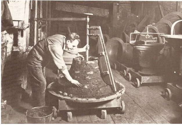
Figure 3-10 Constructing the core of a bell mould
