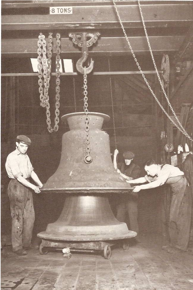
Figure 3-11 Closing core and cope of a bell mould
