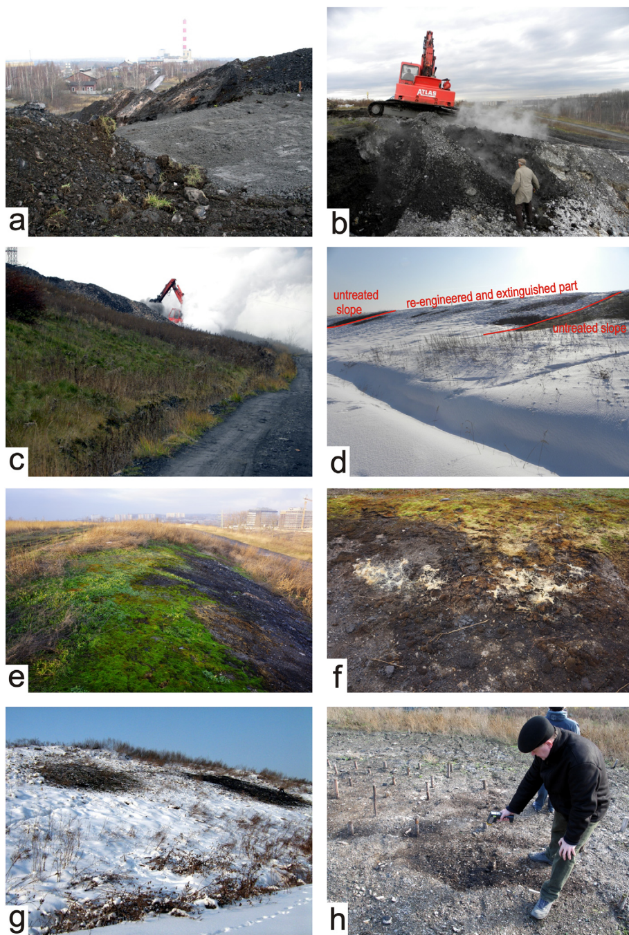
Fig. 2. The Welnowiec municipal waste landfill rehabilitated with coal wastes which heated and ignited. A – Fire-fighting at the eastern part of the northern slope by dug 5-m deep trench filled with fly-ash slurry, December 2008. B – Coal waste of unknown excess thickness used for rehabilitation with higher than planned coal content. C – Fire-fighting in the central part of the northern slope of the dump, November 2009. D – Thermal activity within re-built and extinguished part of the northern slope, appeared on February 2010. Intensification of burning (dark spots) at the borders of extinguished area. E – Burning reaching the easternmost part of the northern slope; heated places promote vegetation growth even in winter (January 2014). F – Exhalative minerals encrusting vents on the dump surface, March 2014. G – Hot spots on the south-eastern slope of the dump: initial thermal activity ~6 m in diameter (left) and vanning activity (right), January 2010. H – Slope stabilization with wooden poles caused intensified thermal activity at the south-eastern slope of the dump. Photos: Justyna Ciesielczuk.
