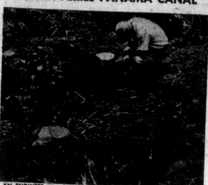
AN ENGINEER examines a deep crack in rock near the Panama Canal. The crack first was discovered in 1938. It was tiny then, but has been getting bigger and bigger. Now plans are being made to remove the rock from face of the hills near the canal, 2,250,000 cubic yards of it, to forestall a possible slide.
