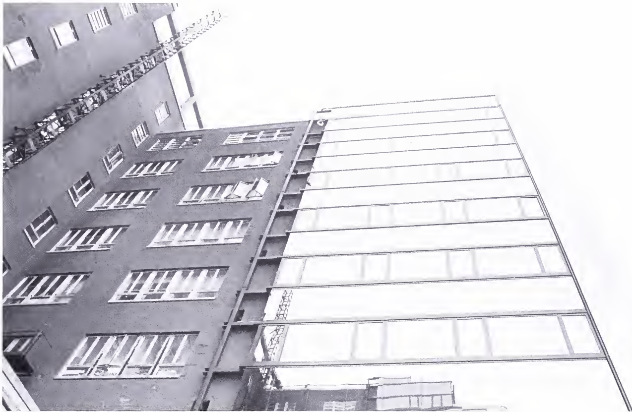
Addition of a new steel and glass exterior continues at Buildings 1 and 2.
