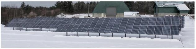
THERE ARE (198) 345 W PANELS MANUFACTURED BY REC SOLAR AND (5) 11.4 KW SOLAREDGE INVERTERS
