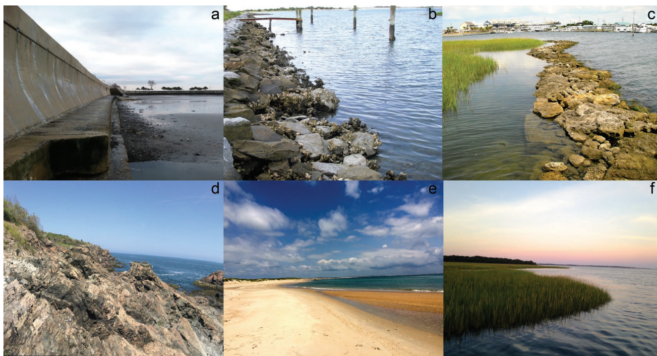
Figure 1. Example of engineered-shore structures: (a) a seawall; (b) riprap revetment; (c) breakwater; and natural shorelines compared in this study: (d) rocky shoreline (granite platforms); (e) soft-sediment shoreline (sand beach); and (f) biogenic shoreline (salt marsh). Rocky shorelines consist of consolidated rocky platforms and/or cobbles and boulders. Soft-sediment shorelines consist of unconsolidated sediments (sands, muds, silts, clays) without intertidal vegetation. Biogenic shorelines can include intertidal and shallow subtidal marsh, mangrove, bivalve or coral reef, or seagrass.
