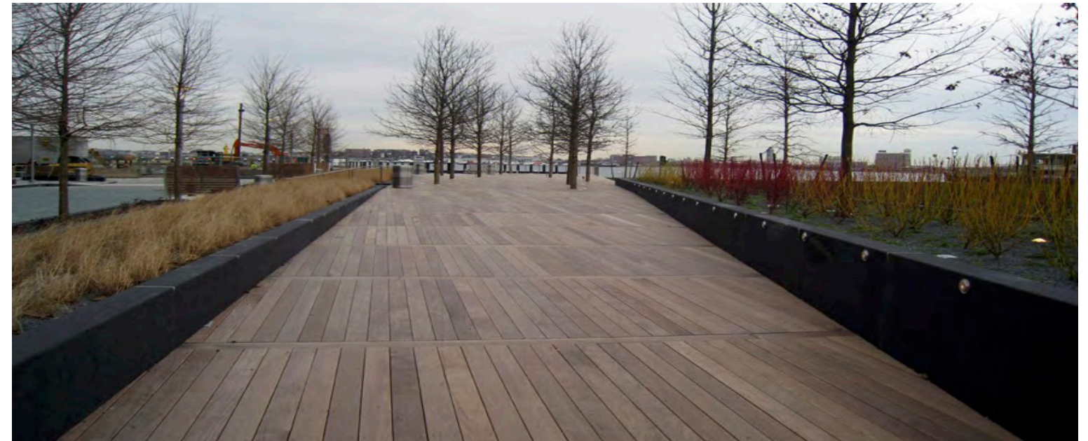
Figure 26: Seaport Public Green, existing conditions hardscaped area.
