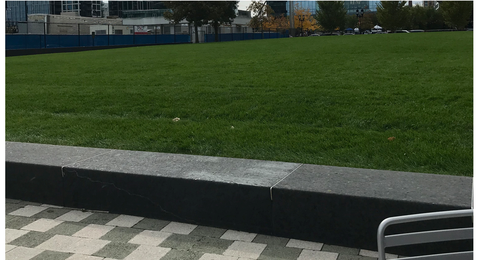
Figure 58: Seaport Public Green in its existing state does not meet the sidewalk at ground-level and has a stone border.
