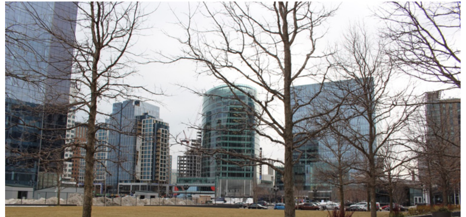
Figure 13: Lack of relationships between spaces in the Seaport and around Seaport Public Green.
