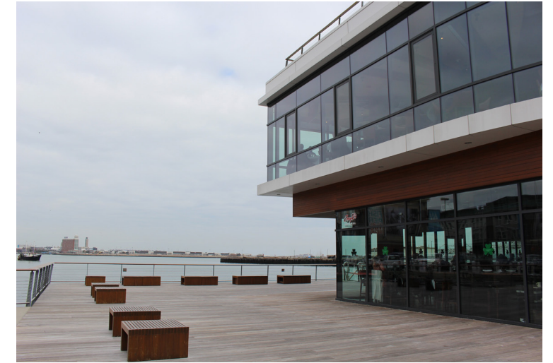
Figures 16: Harborwalk beside Legal Harborside restaurant in the Seaport District.
