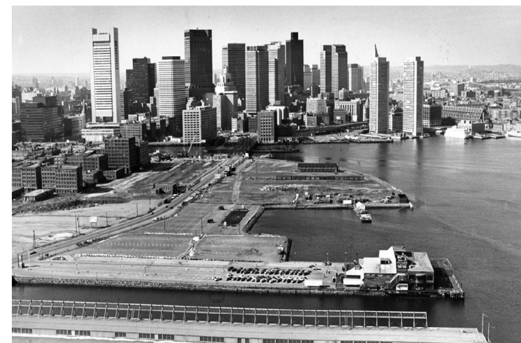
Figure 10: Central Artery cuts off the Seaport District.
