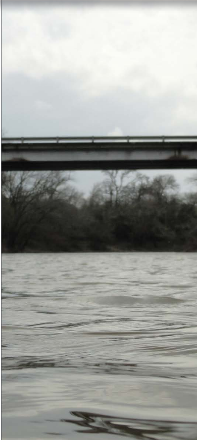
Navasota River at SH 30 near College Station
