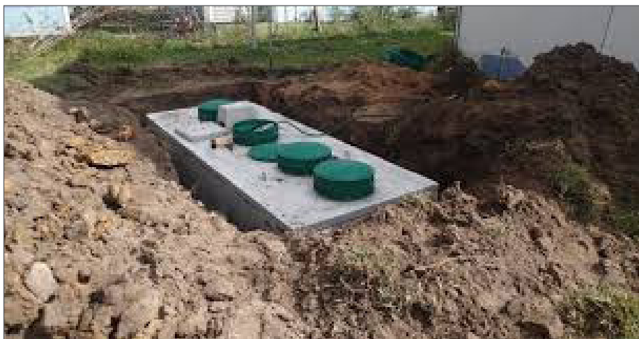
A new OSSF being installed (Texas A&M AgriLife Extension Service)
