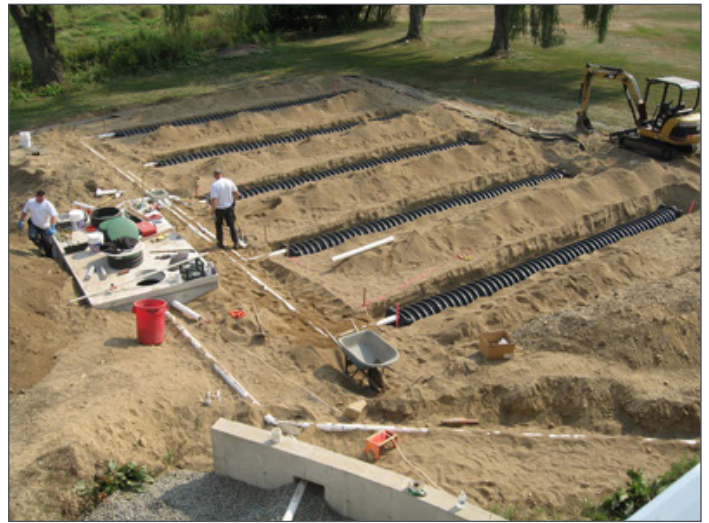
Conventional OSSF installation in progress (omniseptic.com)
