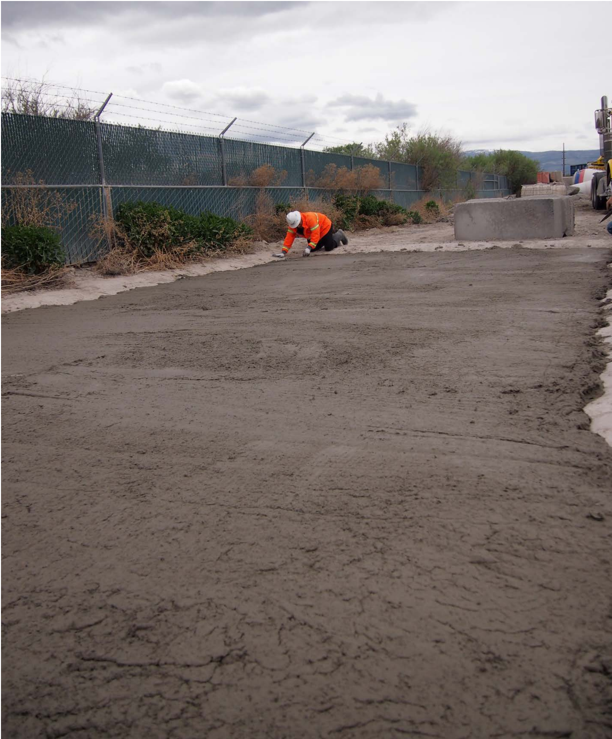
Figure 70 Completed Trial Slab from Trial Batch A.
