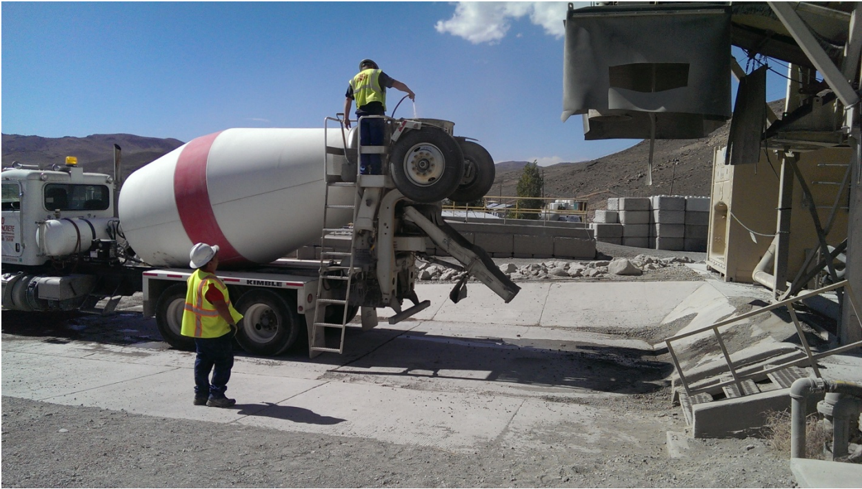
Figure 71 Plant Setup for Truck-Mixed MECC from Trial Batch B.
