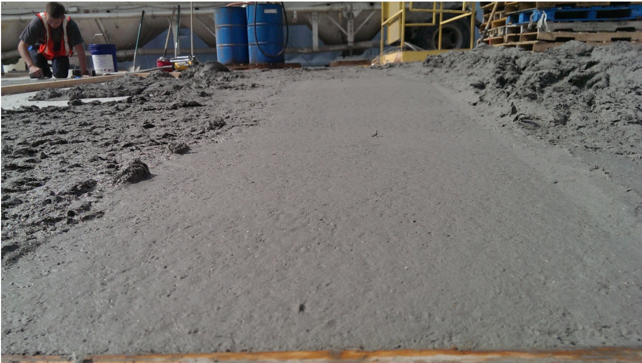
Figure 72 Completed Trial Slab from Trial Batch B.
