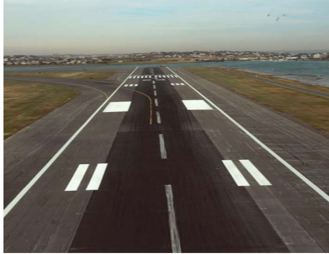
Figure 7 Runway 4R-22L at Logan International Airport (taken on 09-18-07)
