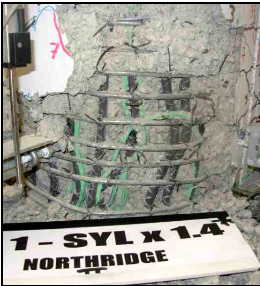
d) Long. Bars Buckling
