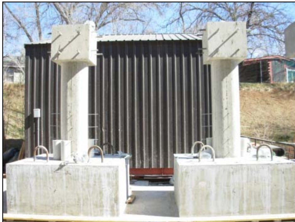
Figure 3-14 Interlocking Columns after Form Removal
