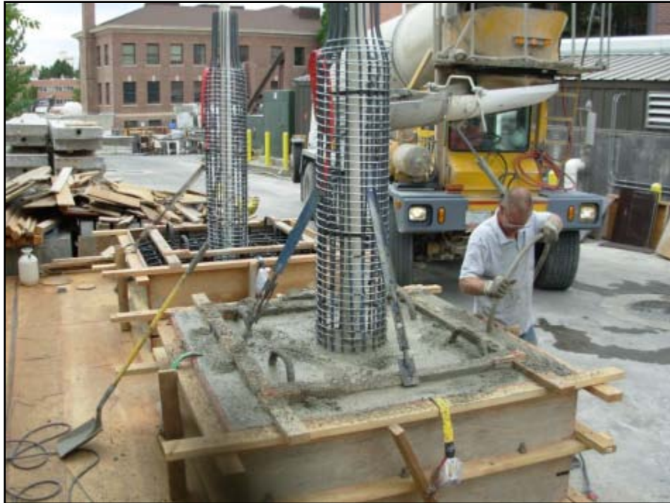
Figure 3-7 Circular Column Footing Concrete Pouring
