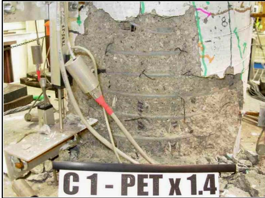
Figure 4-32 Spiral and Longitudinal. Bars visible, Specimen C1
