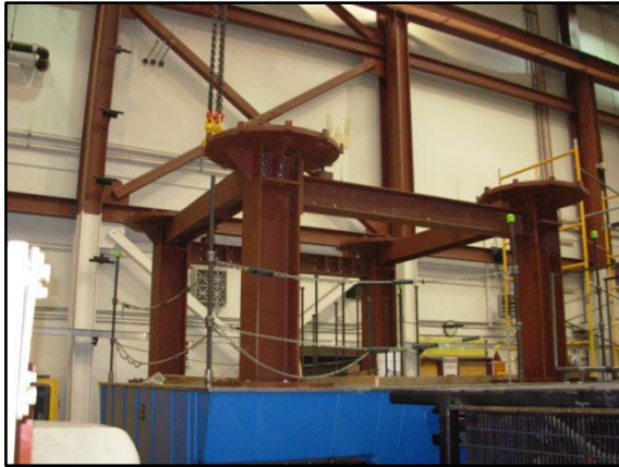
a) Supporting Structure
