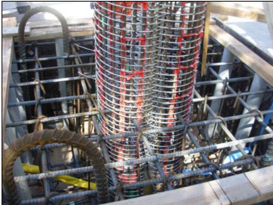
Figure 3-4 Interlocking Column Steel Cage Set on the Footing
