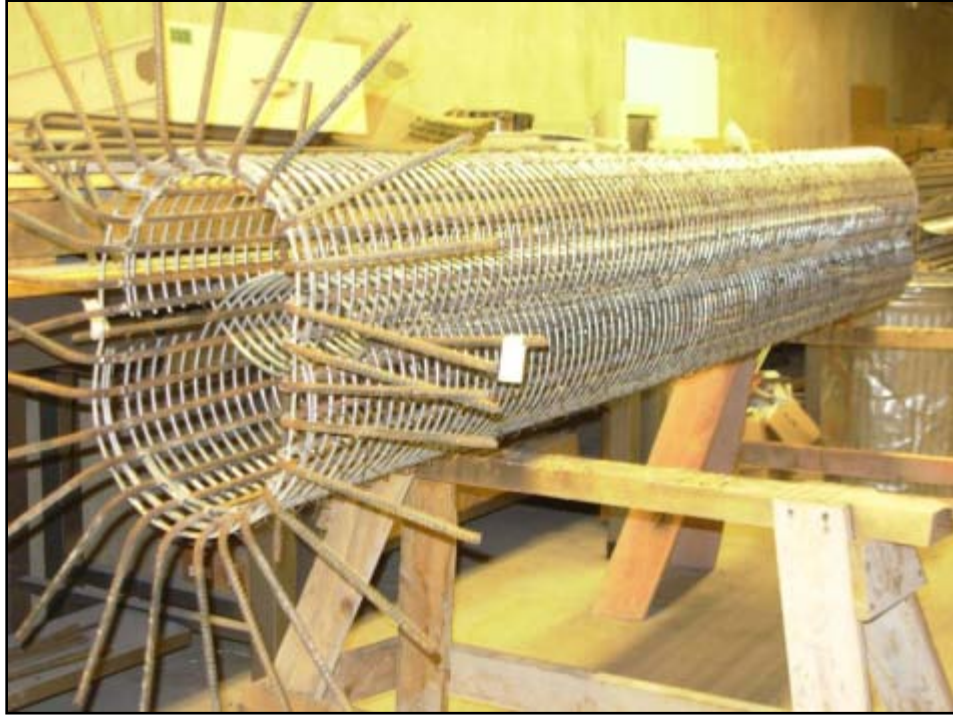
Figure 3-1 Steel Cage for interlocking Column (view from bottom)
