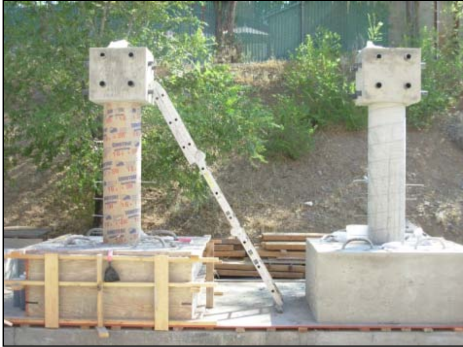
Figure 3-13 Circular Columns after Form Removal
