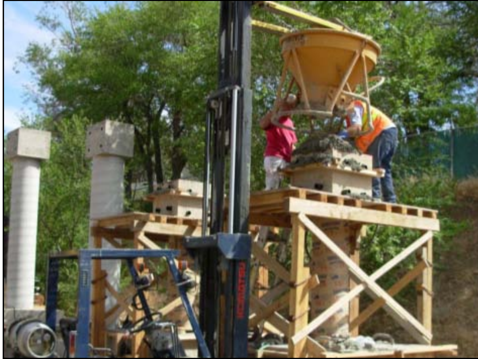
Figure 3-11 Column and top Head Pouring (Circular Specimen)
