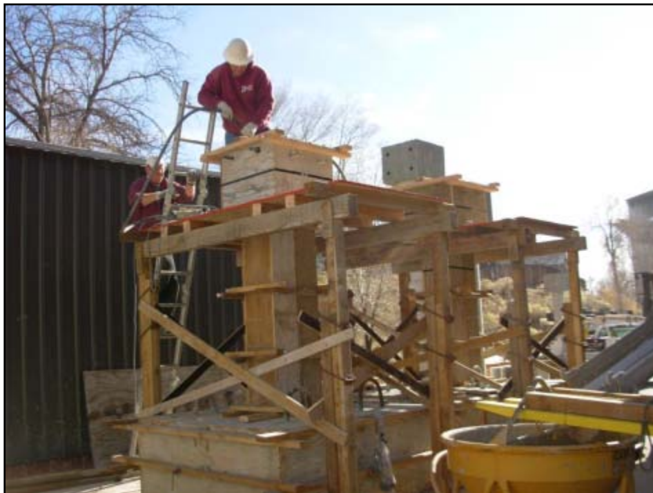
Figure 3-12 Column and top Head Pouring (Interlocking Specimen)
