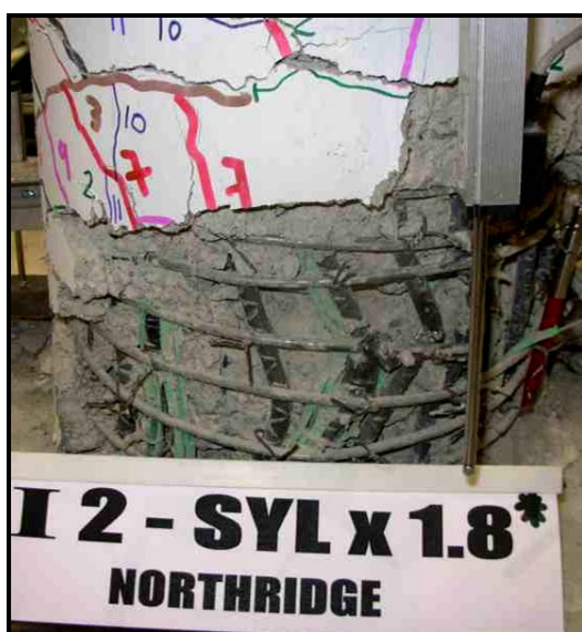
c) Long. Bars Buckling
