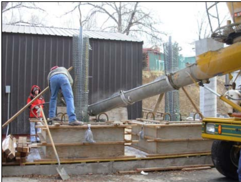
Figure 3-8 Interlocking Column Footing Concrete Pouring
