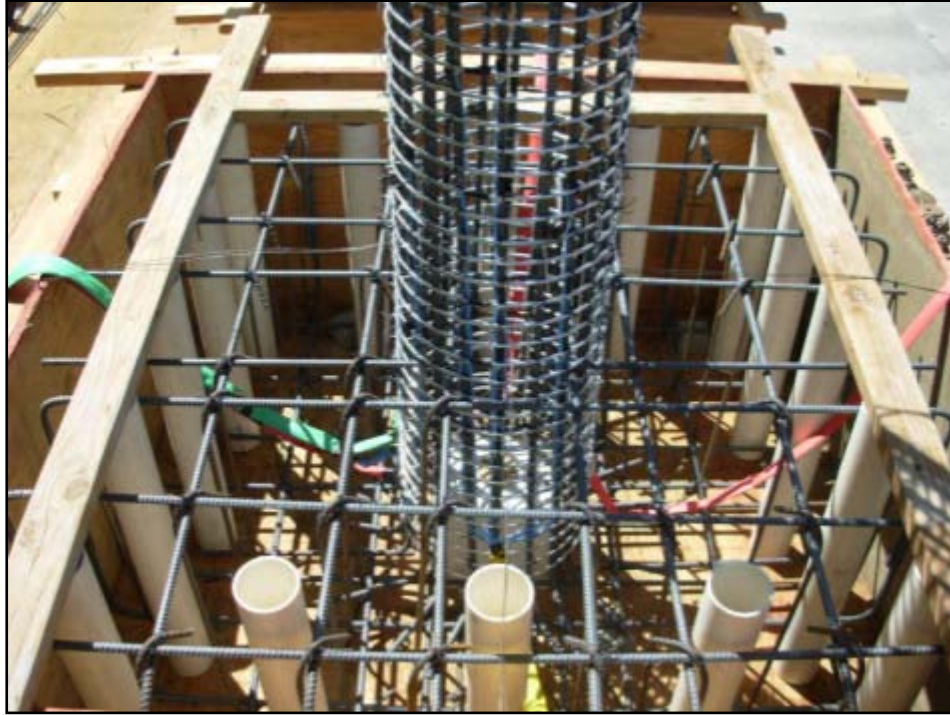
Figure 3-5 Circular Column Footing before Pouring the Concrete
