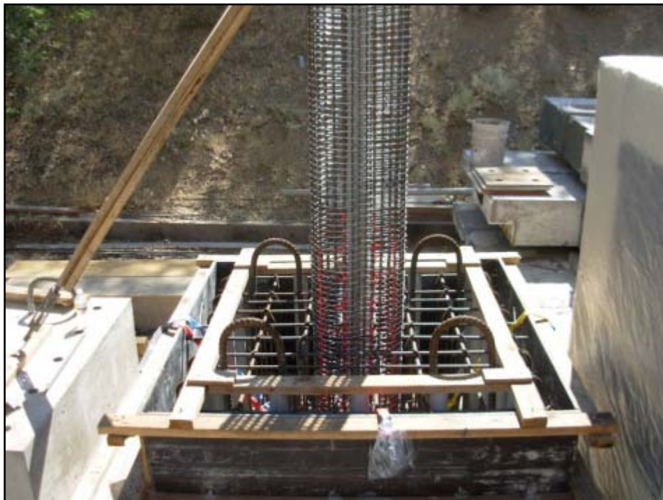
Figure 3-6 Interlocking Column Footing before Pouring the Concrete
