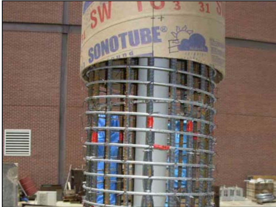
Figure 3-9 Circular Column Formwork
