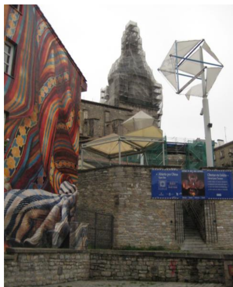
Fig. 1. Restoration of the Catedral de Santa Maria, Vitoria-Gasteiz.
