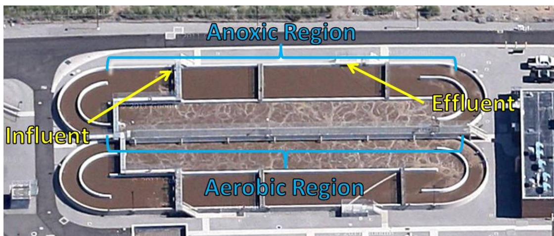
Figure 2-1: Aerial View of Oxidation Ditch at STMWRF
