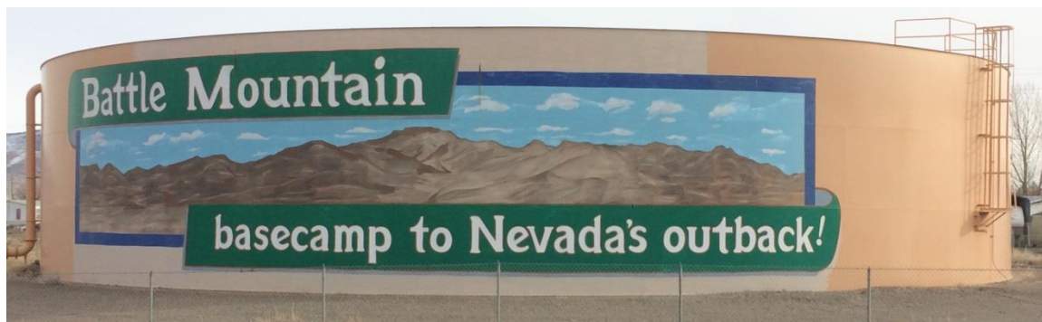
Image 1: Storage Tank in Battle Mountain, Nevada. (Photograph by Samantha Szesciorka, 2016)
