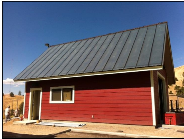
Figure 1-4: DRI Solar Research Laboratory with SBAC Roof
