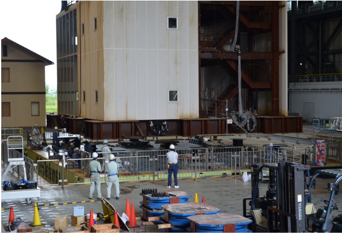
Figure 4-15: Lowering the testbed building over the isolation system
