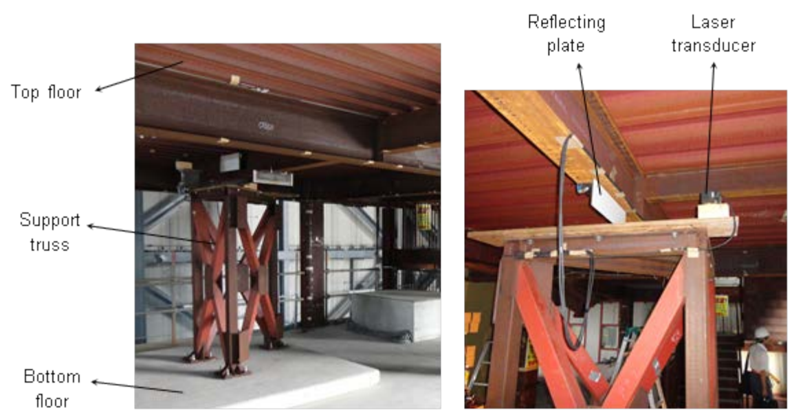
Figure 4-8: Instrumentation for measuring story drift
