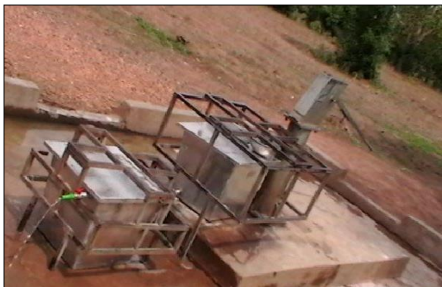
Fig. 1.3. Fluoride adsorption filter attached to a hand-pump well in rural northern Ghana (World Vision, 2014)
