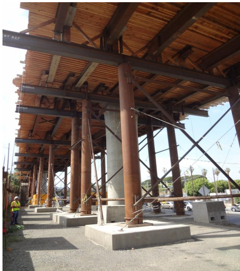
Figure 9-4 Falsework in Bridge 4
