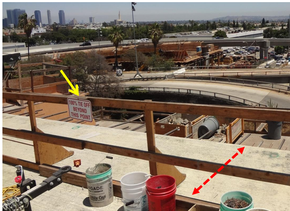
Figure 3-15 Tie-off point in Bridge 4
