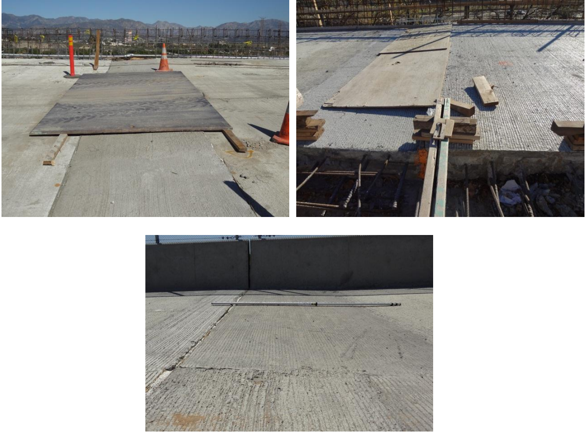
Figure 1-5 Hinge curl during construction
