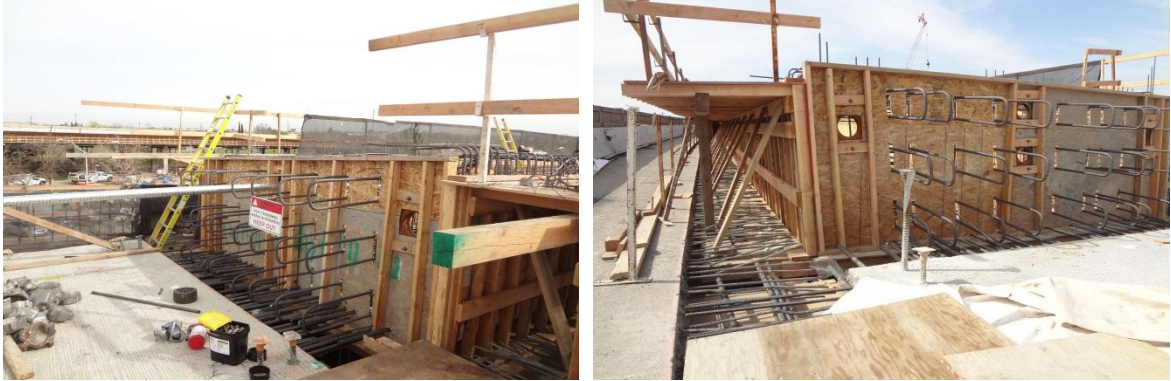
Figure 2-53 Drop-in span construction views at Closure 1 and 2
