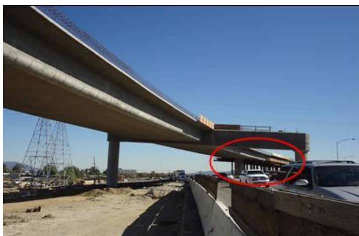
Figure 4-23 Partial falsework removal in Frame 2 on Day 148
