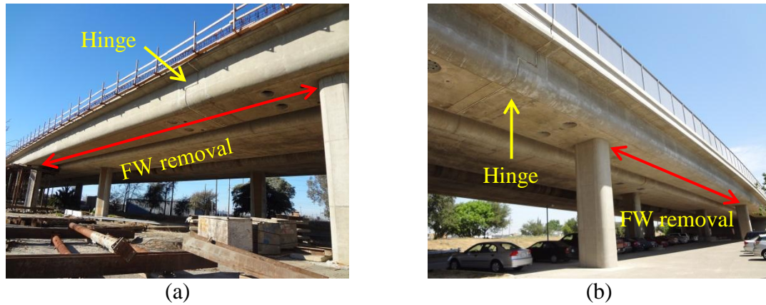
Figure 2-12 Falsework removal in: (a) hinge span; and (b) adjacent span
