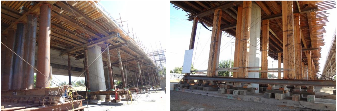
(a) (b) Figure 2-8 Falsework posts: (a) Steel posts; and (b) Timber posts
