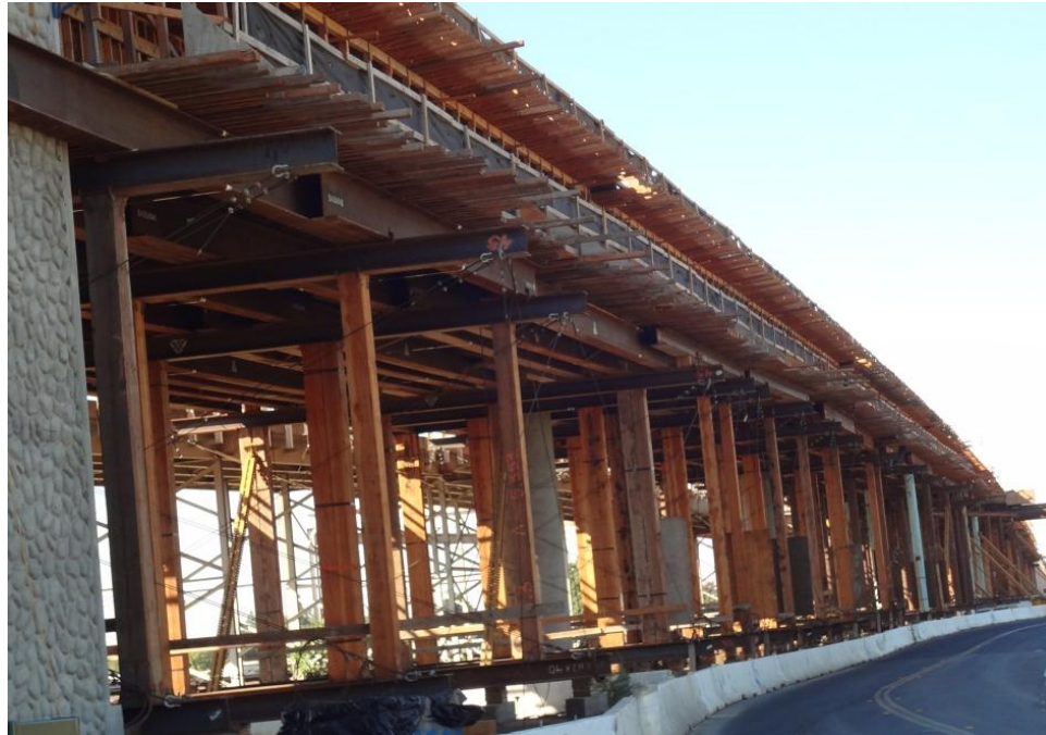
Figure 1-1 Bridge falsework, Del Paso Park Overhead, Sacramento
