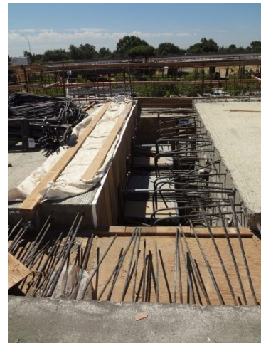
Figure 1-4 Construction of in-span hinges in CIP/PS box girder bridge
