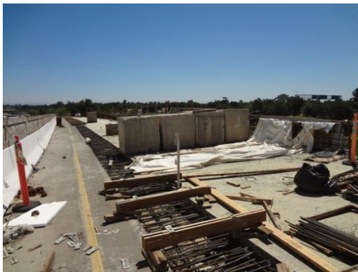
Figure 1-8 Hinge curl repair by loading the short cantilever of an in-span hinge in Del Paso Park Overhead, Sacramento
