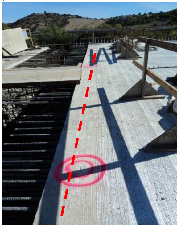
Figure 3-6: (a) Station marking process; (b) Typical station; (c) Typical transverse gridline at the hinge
