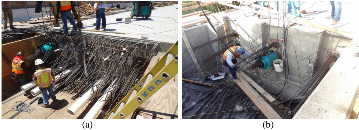
Figure 2-13 Prestressing process at: (a) Hinge; (b) Abutment
