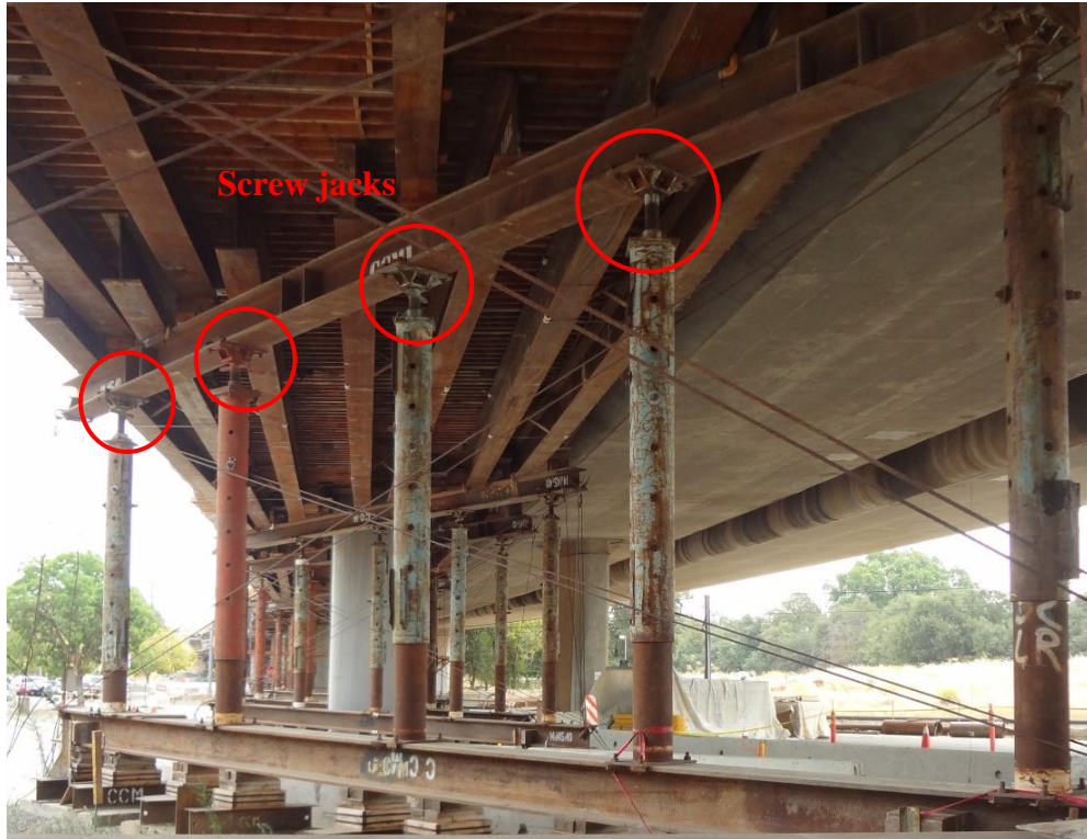
Figure 1-9 Adjustable falsework posts, Del Paso Park Overhead, Sacramento
