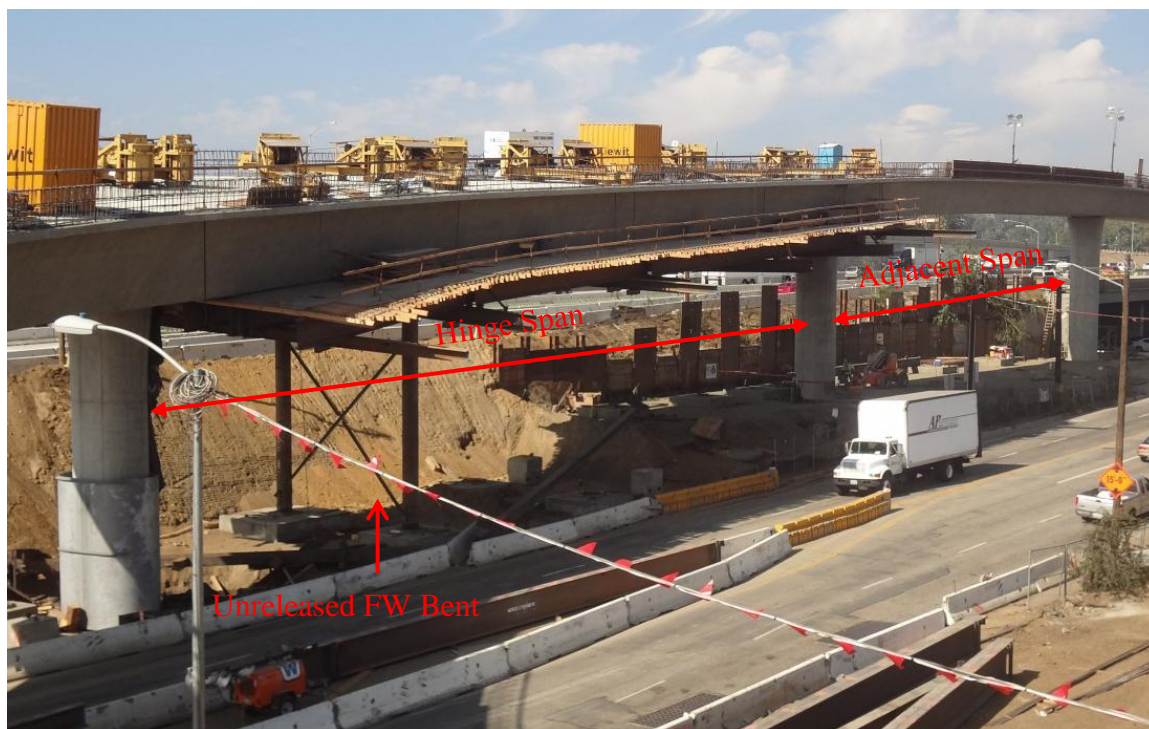
Figure 8-38 Partial load transfer at H, Bridge 4
