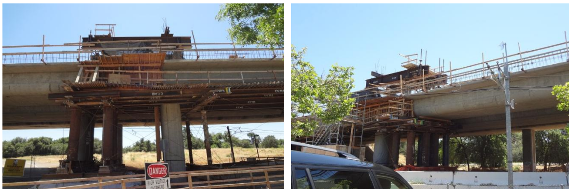
Figure 2-56 End supports of the drop-in span
