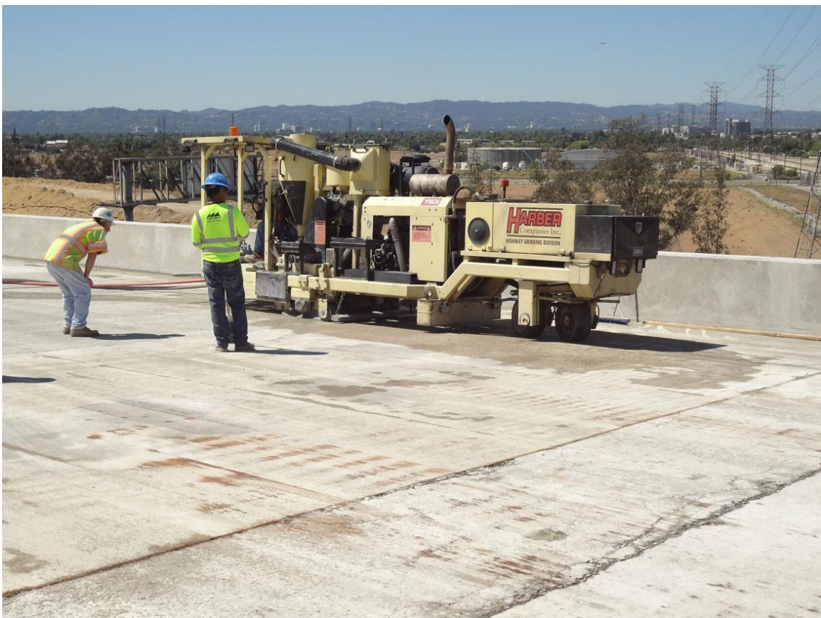
Figure 2-5 Deck grinding at the hinge area using a grinding machine
