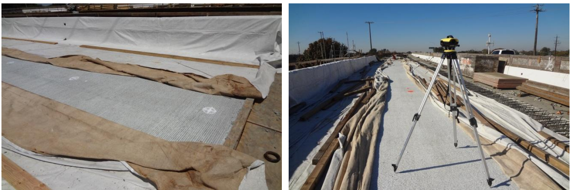
Figure 3-2 Deck surface partial reveal for stations marking during concrete curing
