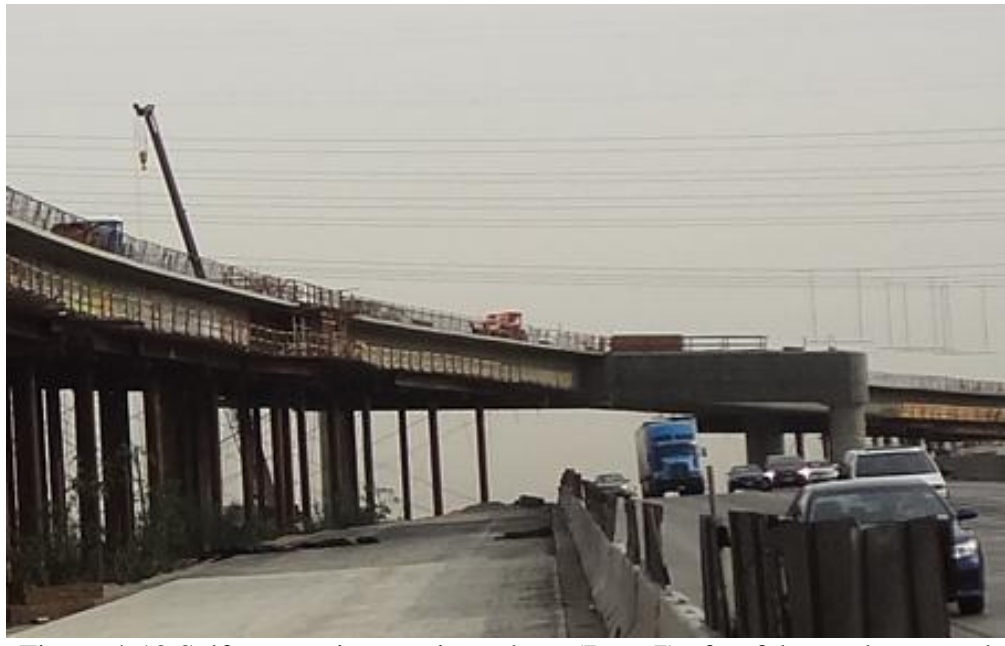
Figure 4-12 Self-supporting outrigger bent (Bent 7) after falsework removal
