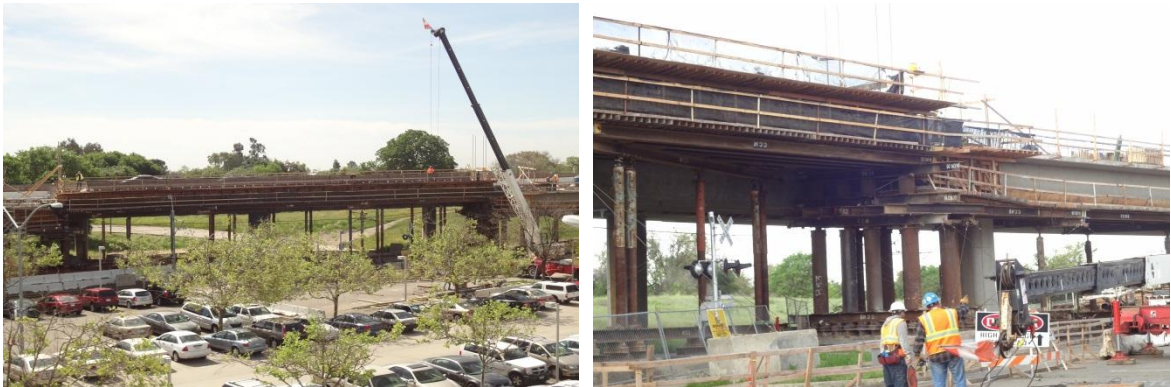
Figure 2-54 Drop-in span falsework
