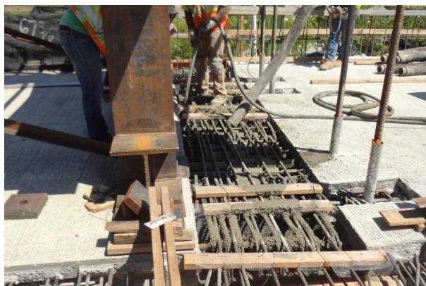
Figure 2-48 Concrete pouring of Closure 1
