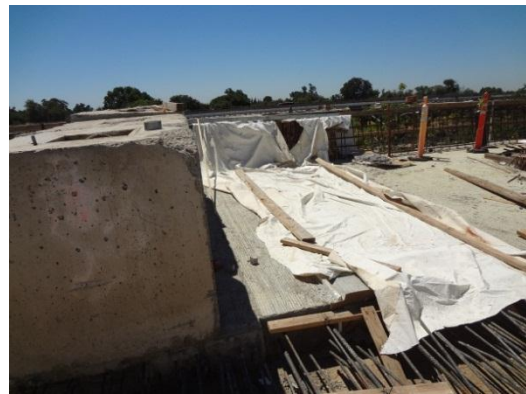
Figure 1-8 Hinge curl repair by loading the short cantilever of an in-span hinge in Del Paso Park Overhead, Sacramento
