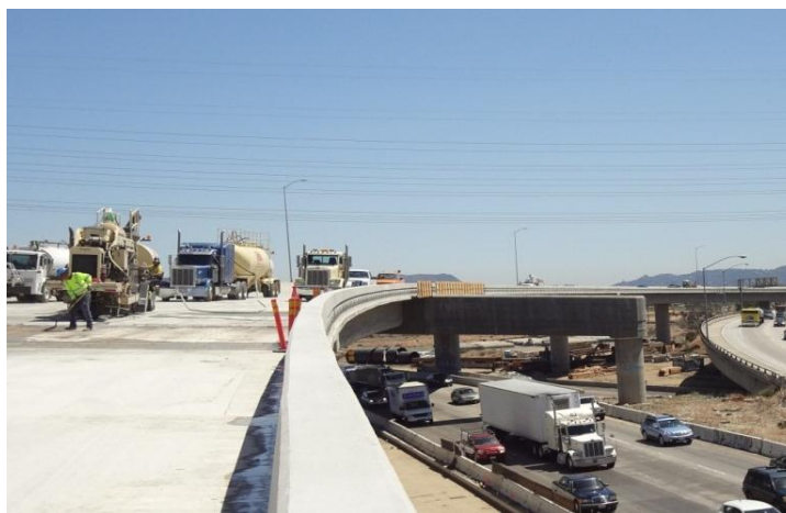
Figure 4-24 Complete falsework removal in Frame 2
