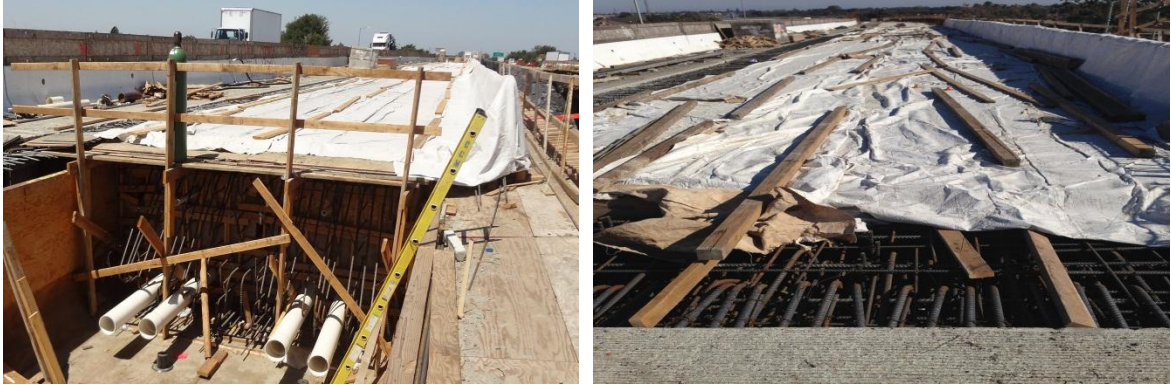
Figure 3-1 Moisture retaining blankets for concrete curing
