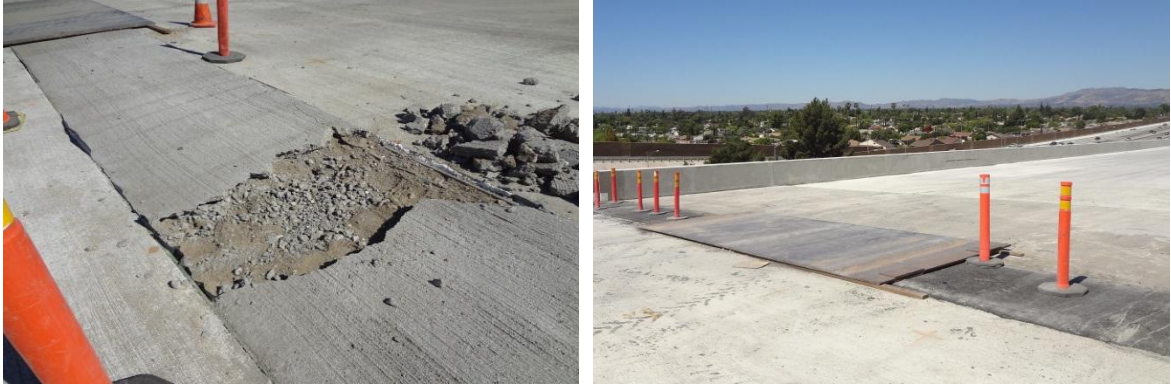
Figure 2-4 Temporary fill of joint seal assembly blockout void
