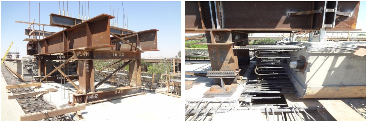
Figure 2-55 Steel frames holding the drop-in span
