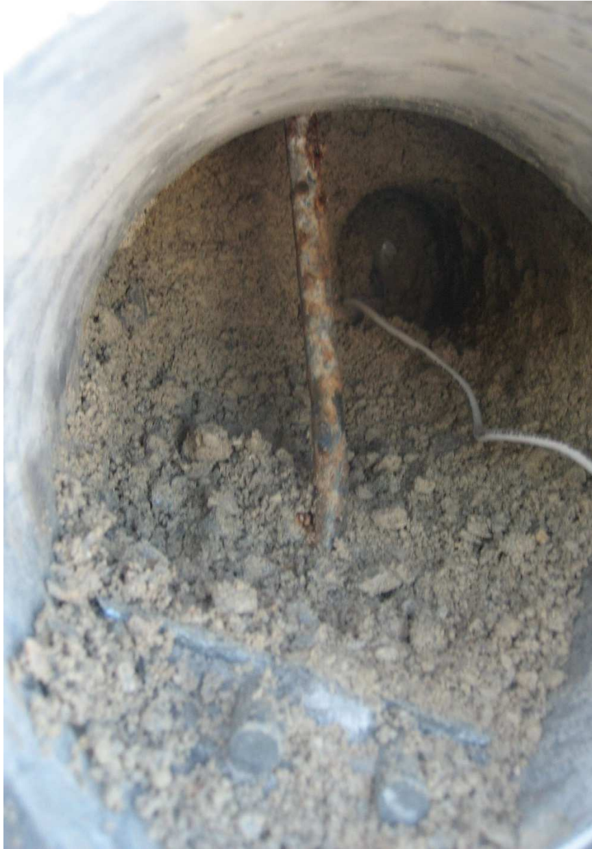
Figure 3-19: I-15/ Lamb Blvd. in-service reinforcement WA-SA-E2
