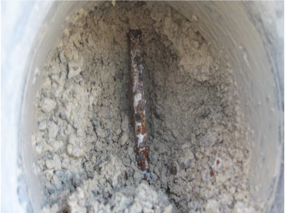
Figure 3-18: I-15/ Lamb Blvd. in-service reinforcement WA-SA-E1
