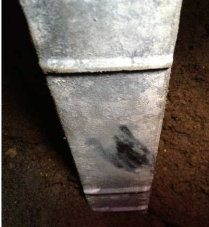
Figure 0-2: In-service galvanized reinforcement, a layer zinc carbonate can be seen along the surface. (ALT US 95 and ALT US 50, W1-SB-E1)
