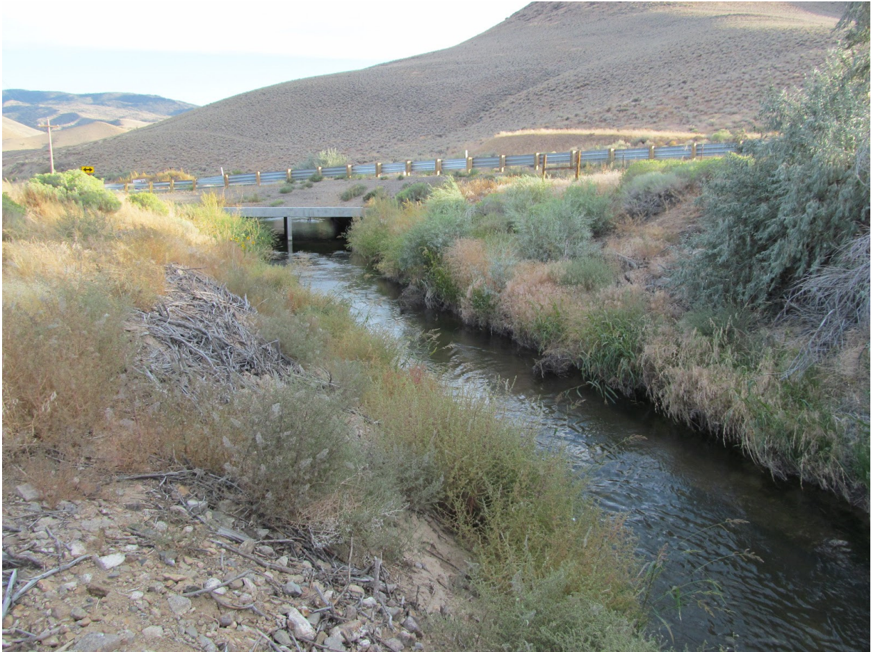
Figure 37: Irrigation ditch, Smith Valley, Nevada. One of many ditches used throughout the valley for widespread diversion of the Walker River for agricultural irrigation. Photo taken at 5:15pm 8/26/16.
