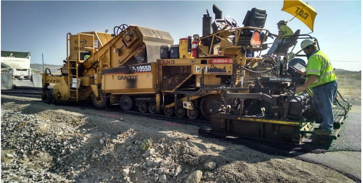
Figure 9. 5. Picture of the Windrow Lifter and Paver
