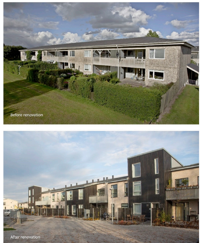
Fig. 4. The Case study building before and after renovation. After renovation the building features larger windows and shallow balconies to provide more daylight in the dwellings.
